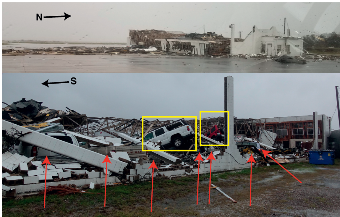
Fig. 7. Damage to buildings and cars (yellow boxes) near the DOW8 location at the Aransas County Airport (Wurman and Kosiba 2018).
