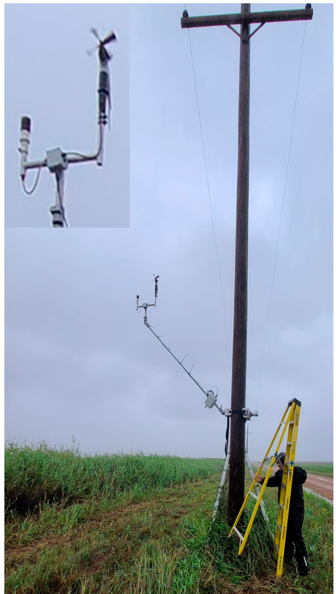
Fig. 11. FARM POLENET unit being deployed on power pole during Hurricane Delta (2020).
