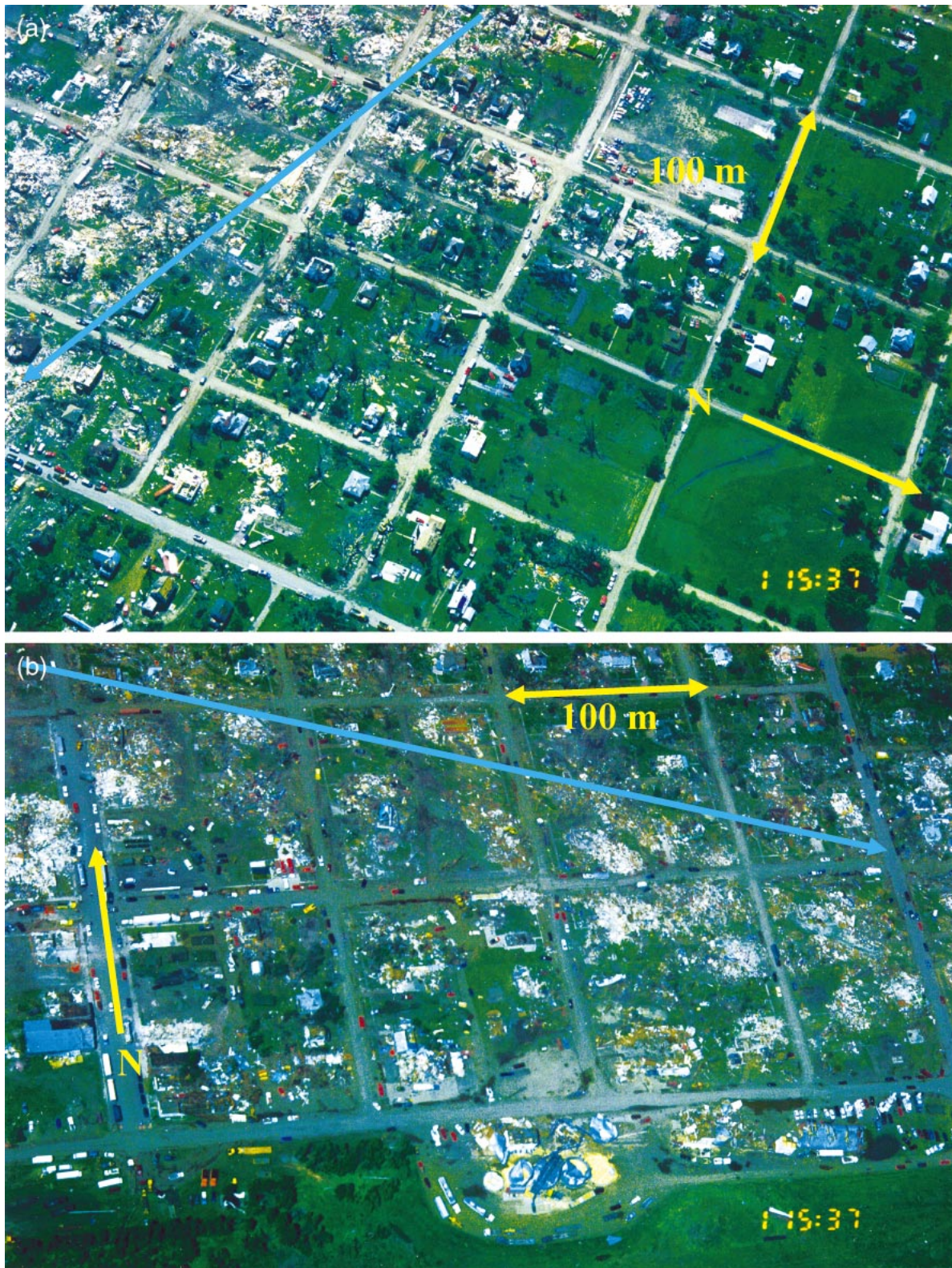
FIG. 3. Aerial photographs of the tornado damage in Spencer showing (a) the north side and (b) the south side of the damage track. The cyan arrow represents the interpolated path of the Doppler velocity couplet center based on DOW radar data (courtesy of B. Smith).
